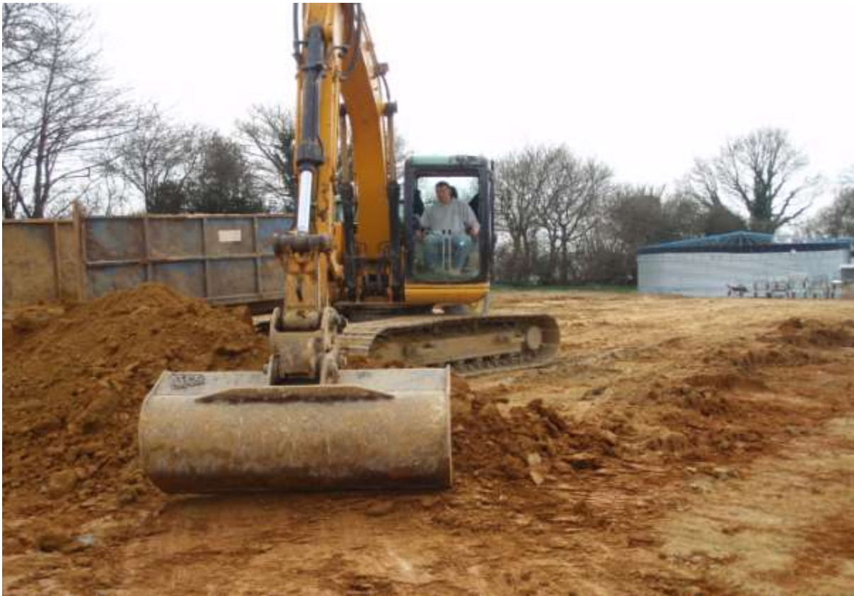
Plate 4. The site showing the slope being removed in spits (looking south)
