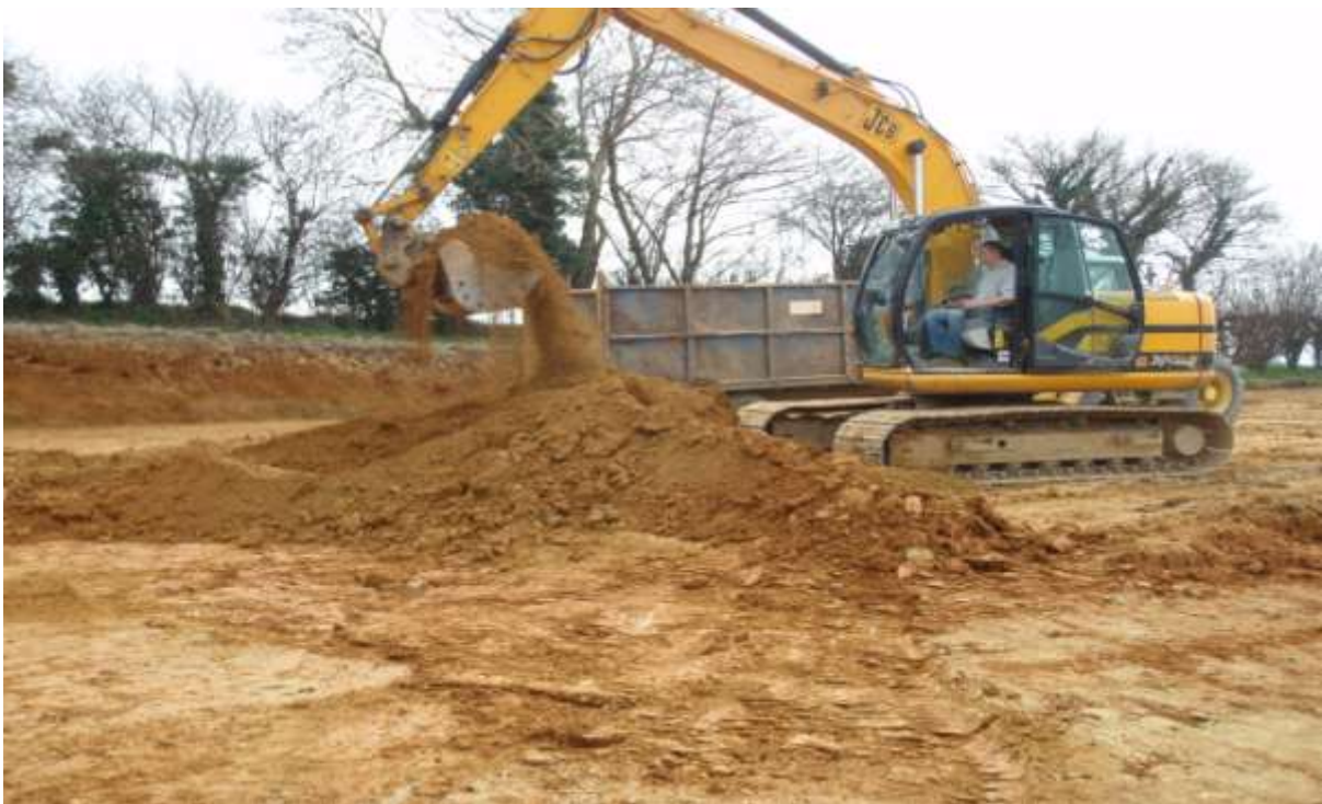
Plate 5. The site showing removal of slope with ditching bucket (looking south-east)
