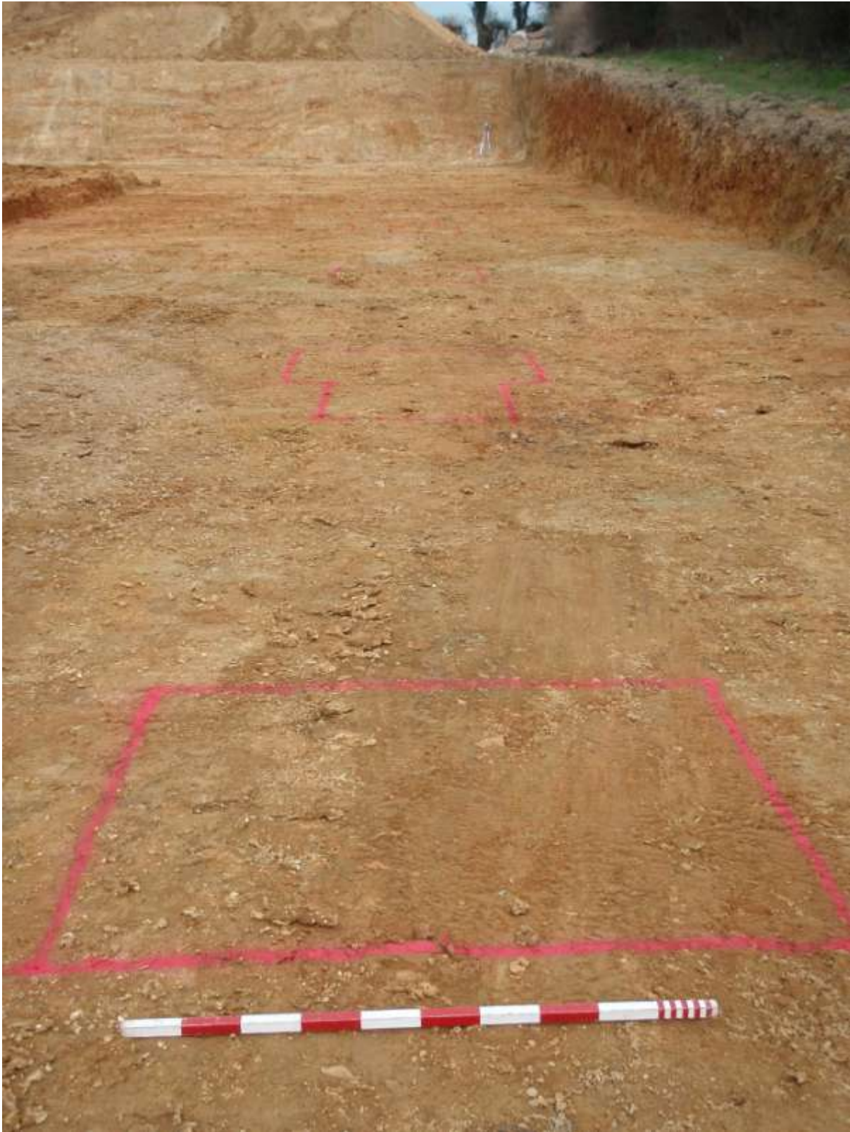
Plate 7. The site showing layout of projected concrete post pads (looking north-east)
