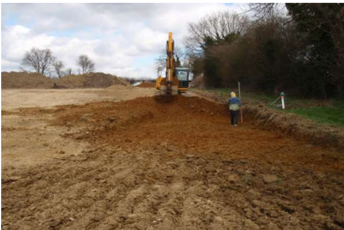
Plate 3. The site showing ground workers removing the slope (looking north-east)
