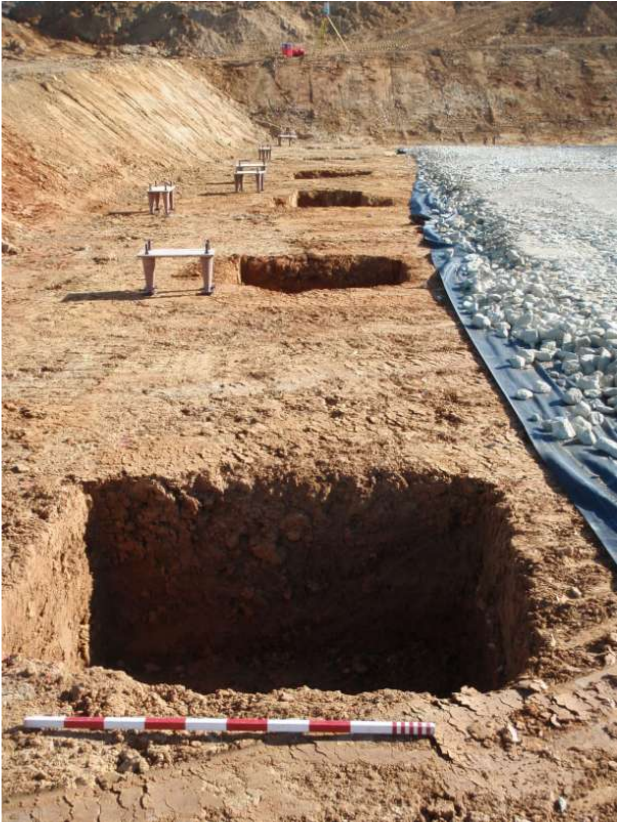
Plate 8. The site showing completed excavation of post pads (looking south-east)
